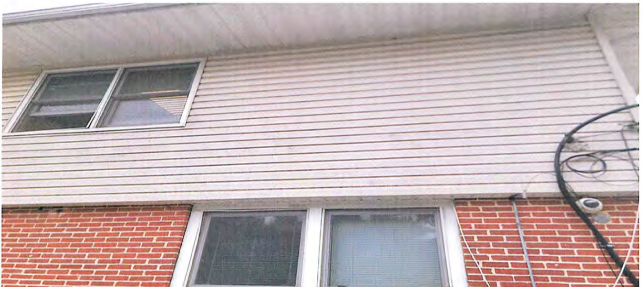
Rear back building with exterior mold
